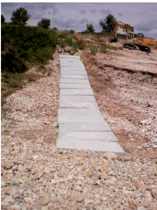
Concrete slab work site
